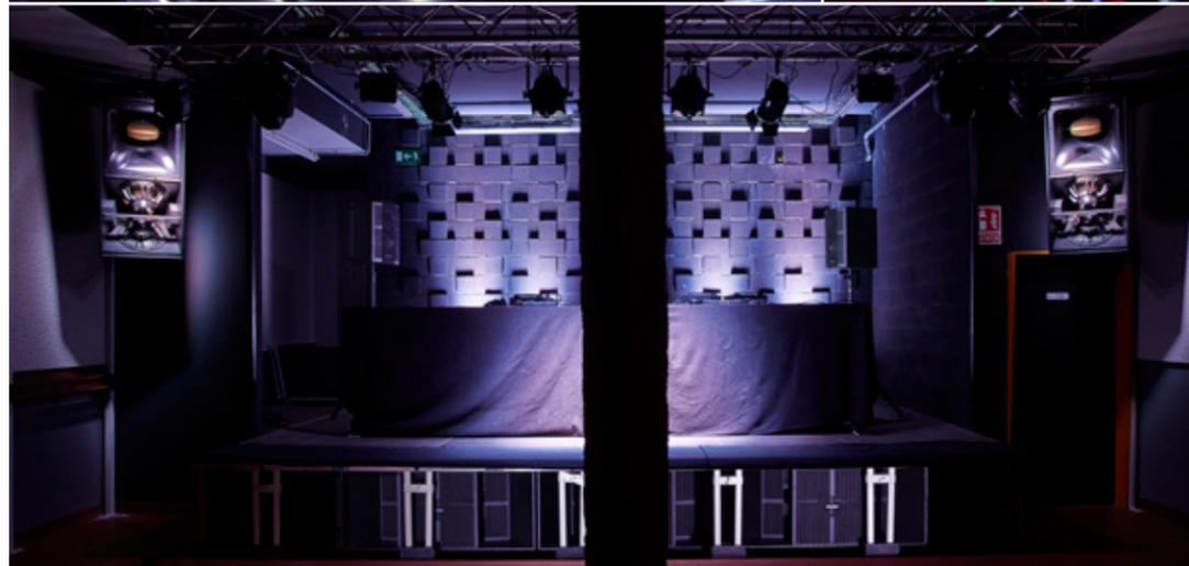
Services installed a four-point system with XY-3B three-way full range speakers either side of the stage, XY-2 mid-high speakers at the rear of the room and a trio of XY-218HS dual 18-inch horn-loaded subwoofers supplying powerful low-end. Using presets on the mixer, the club's management can easily switch to a live gig configuration which uses only the boxes at the front.
